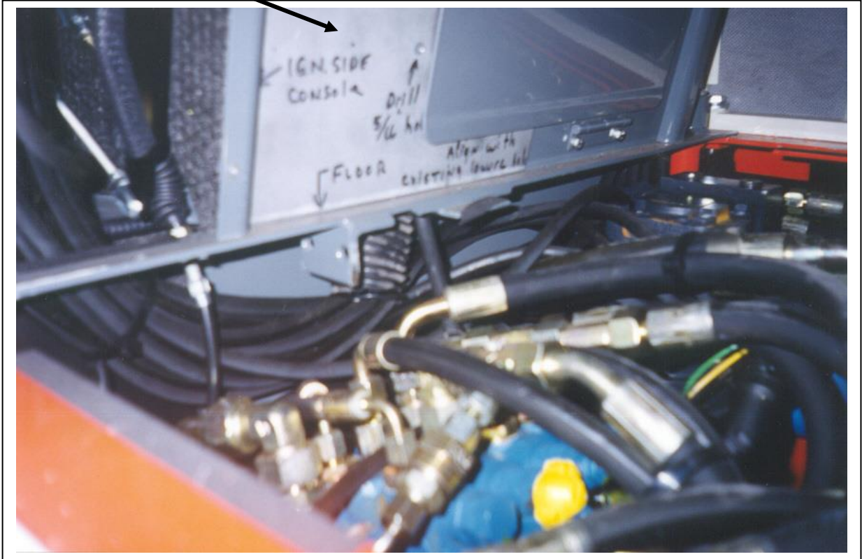
Front mounting hole template in place
